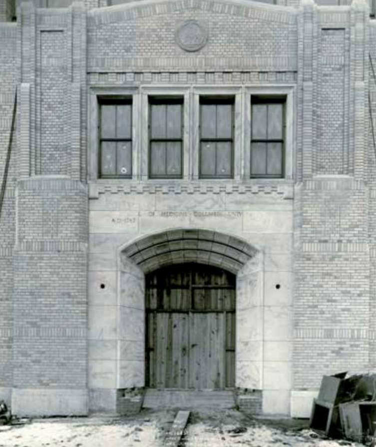
The entrance to the P&S building under construction, Jan. 3, 1927
