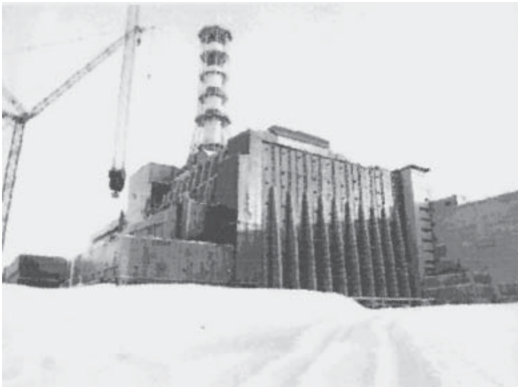
To contain further contamination, this “shelter” was constructed over the nuclear reactor site.
